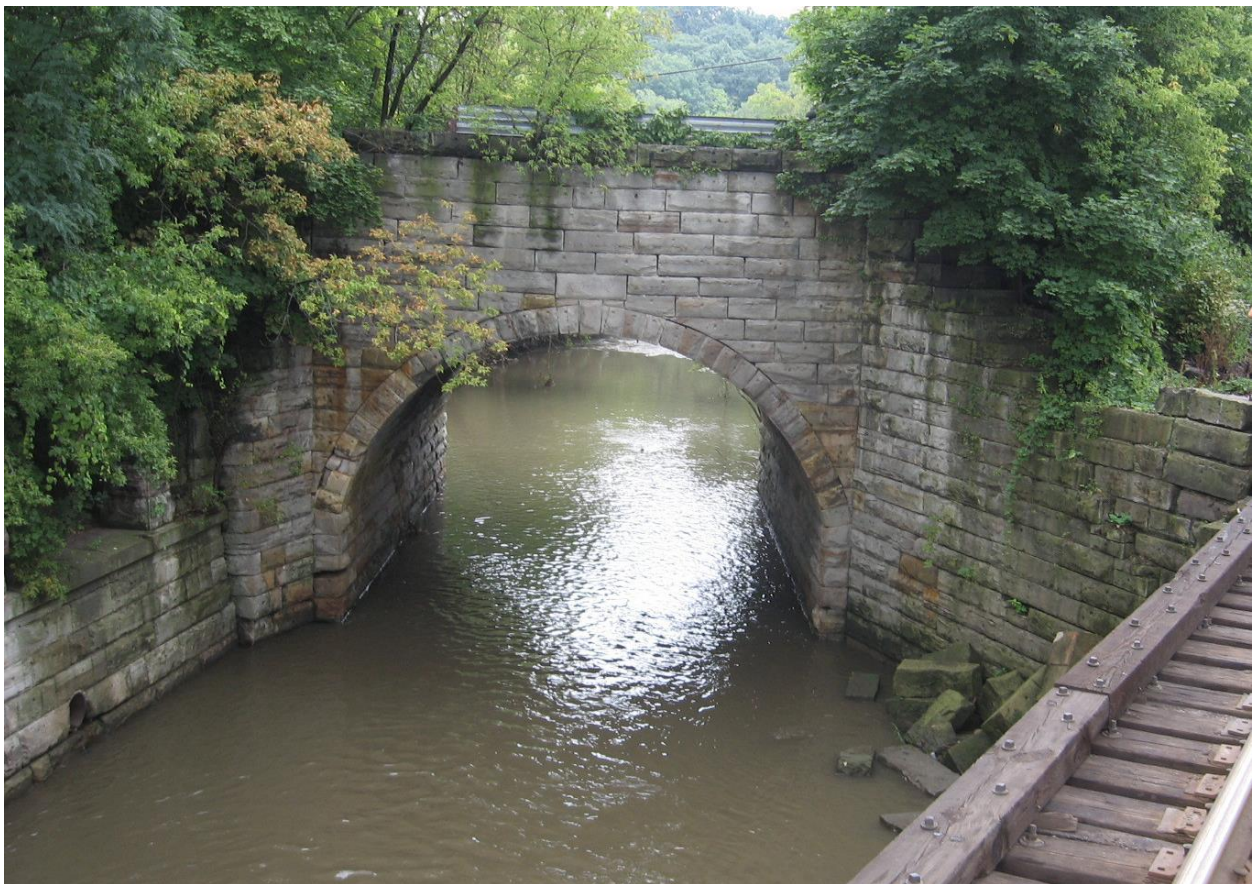
Figure 1. Old Pear Road Bridge over Big Creek.
