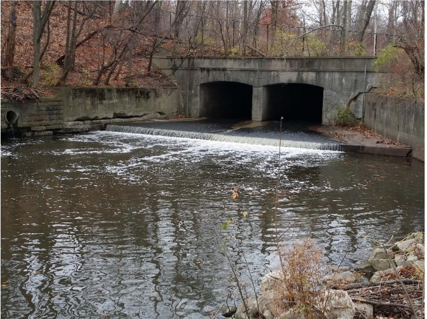
Figure 11. Double barrel culvert of Big Creek at the Cleveland Metroparks Zoo.
