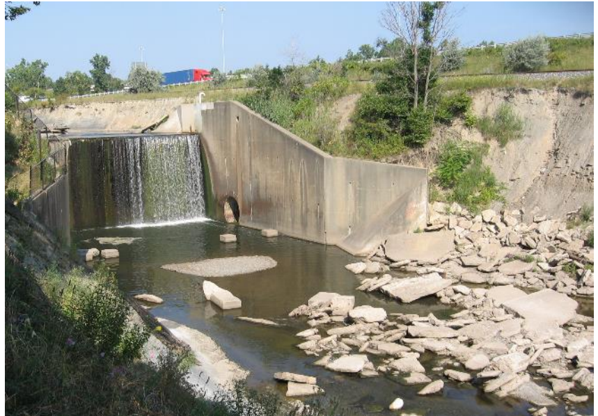
Figure 14. Big Creek drop structure along I-71.
